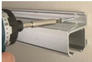
Step 1: Install wall-mount track.
