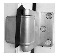
3. Pull the door closed and gently pull on the tool at the same time. This motion should disengage the latch arm as shown below.
