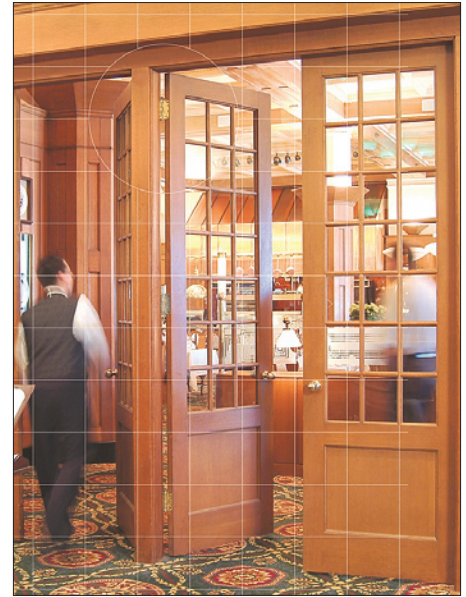
Architectural grade hinges, Station Grill - Union Station, St. Louis, MO
